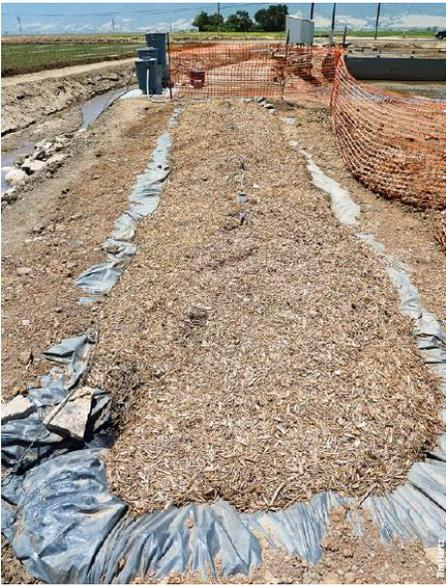
**FIGURE 5. COMPLETED DENITRIFICATION WOODCHIP BIOREACTOR. CREDIT: TIM HARTZ (HARTZ ET AL. 2017).**
