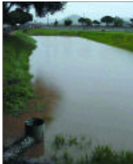
Sediment Basins capture soil and slow storm and irrigation runoff.
