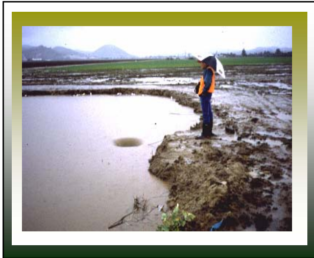
NRCs Engineer observes weir flow in a storm water detention basin.
