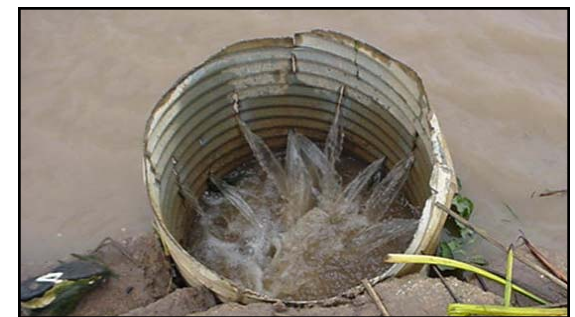
Water entering slotted pipe riser.
